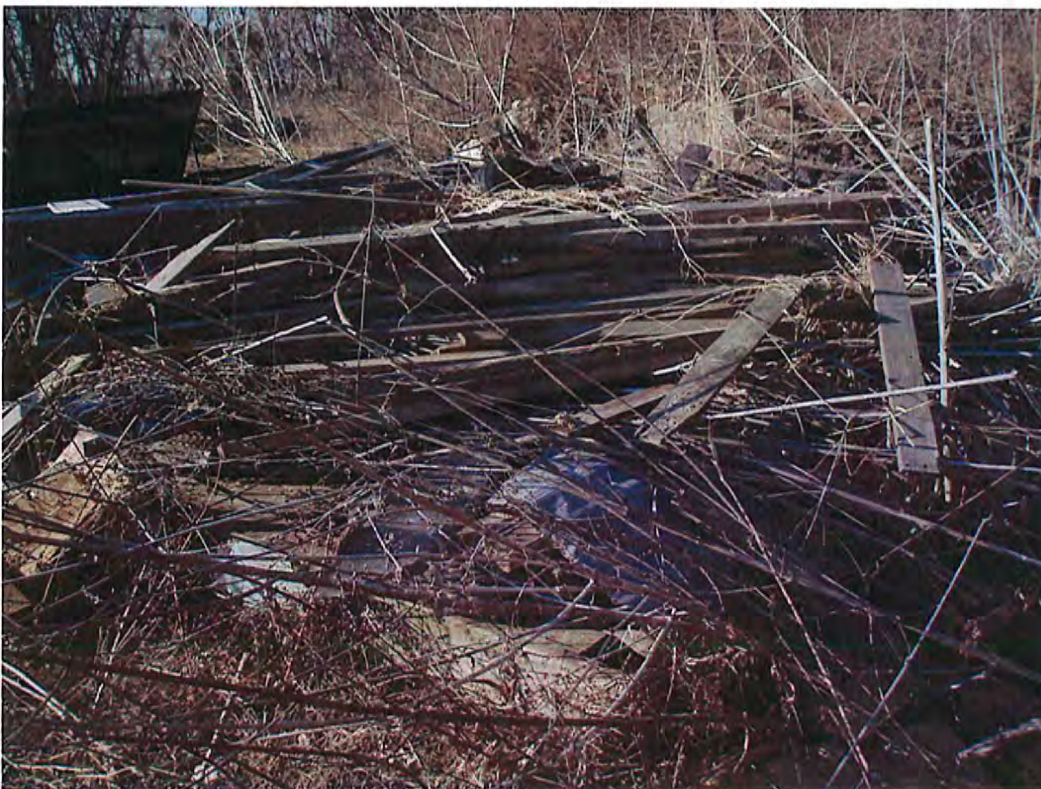
Date: 1/30/2015 Time: 3:29 P.M. Direction: north Photo by: S. Williams Exposure #: 018 Comments: demolition debris
